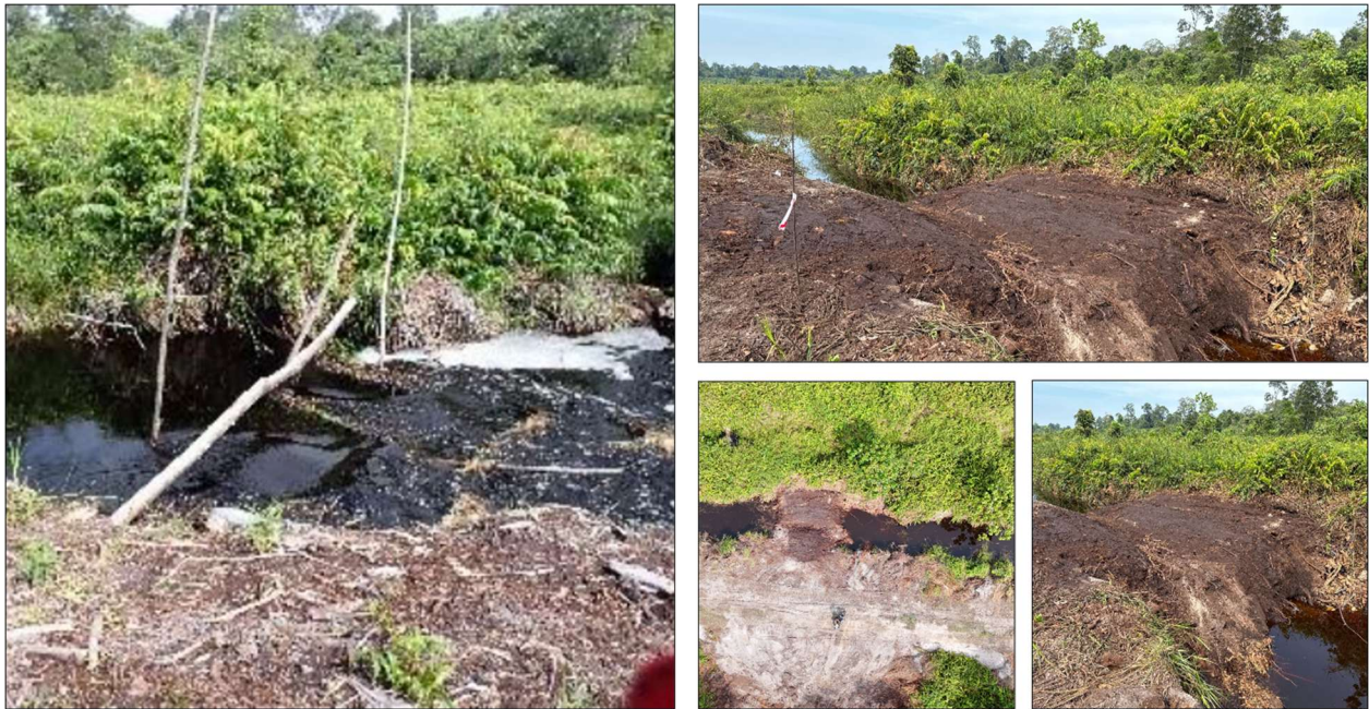
Figure 14: Pre- (left) and post-(right) canal blocking by peat compaction in Tanjung Medang, Pekan FR (Canal Block ID: CB_PKN046)
